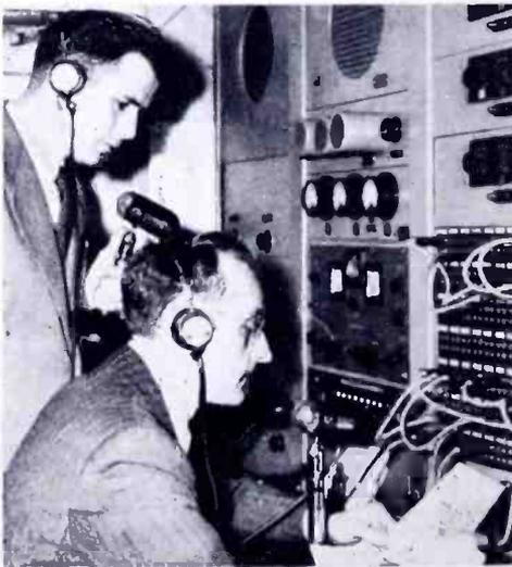
Fig. 2 — Early program control board showing jack field in use for program switching.
