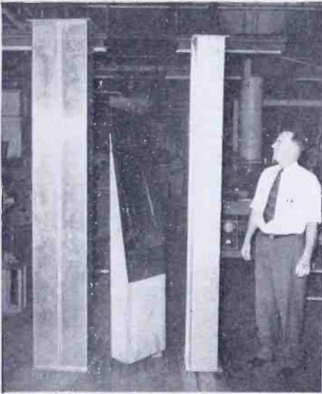
Fig. 16—Straight wave-guide section  $7\frac{1}{2} \times 15$  inches.
